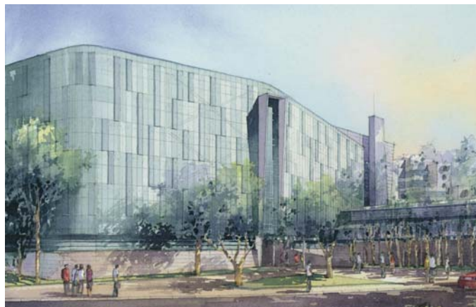
The building design is optimized for wireless communications. Large "propagation windows" rendered in clear glazing, and insulated curtainwall material and Trespa paneling were chosen for the building exterior to allow transmission of line-of-sight communication signals.
